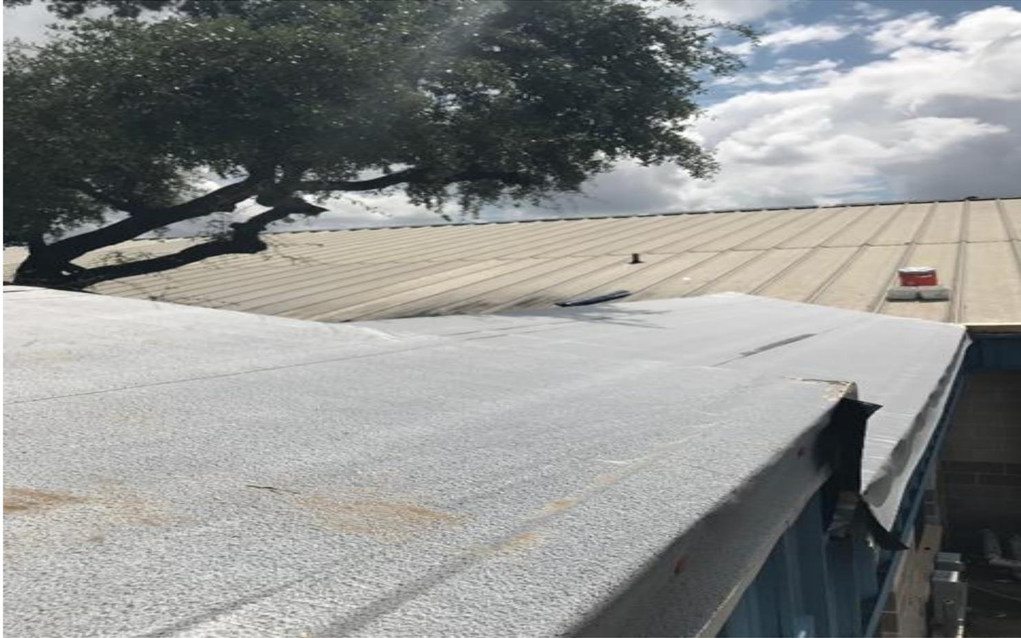
Description: Installation of Roof Hugger System and Insulation on Corridors G5 and G6
