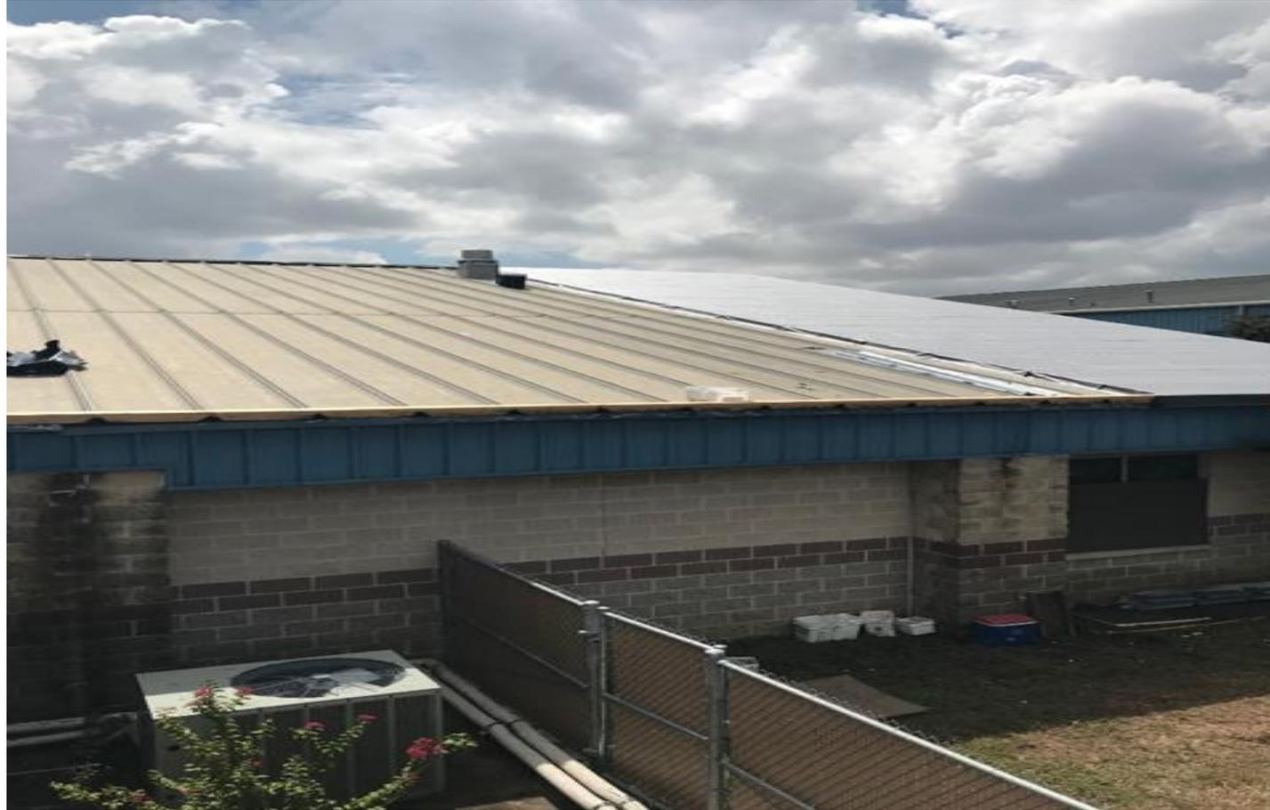
Description: Installation of Roof Hugger System and Insulation on Building B (Cafeteria)
